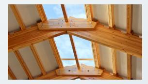
ABF researchers are developing technical information to enable increased use of engineered wood products such as laminated veneer lumber (shown in photo) in wall, roof and floor systems.
