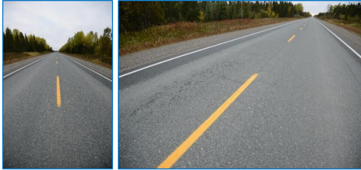
Figure 2. Representative photographs of 12-year-old, PET fiber-modified Cold Lake asphalt Section 9 on Highway 655 north of Timmins, Ontario (base asphalt is 300/400 pen or PG 46-34).
