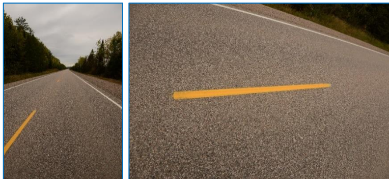
Figure 3. Representative photographs of an 8-year-old, 10 km long contract on Trans-Canada Highway 17 north of Algonquin Park constructed with base asphalt cement produced by a Montreal, Quebec refinery using crude oil derived from Alberta oil sands.
