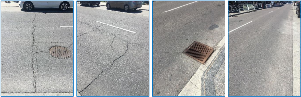
Figure 4. Representative photographs of a 10-year-old stretch of Princess Street in downtown Kingston, Ontario (two left images) and an adjacent 9-year-old stretch (two right images).
