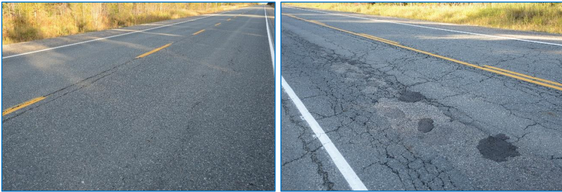
Figure 1. Comparison of best Section 1 (left) and worst Section 4 (right) performing PG 64-34 binders on Highway 655. Note: Construction was completed in late 2003 and photographs taken 16 years later.
