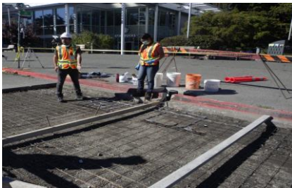
e) Joints for three bus pads
