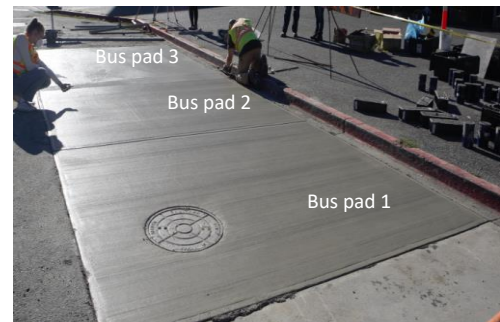
h) Final shape of three bus pads
