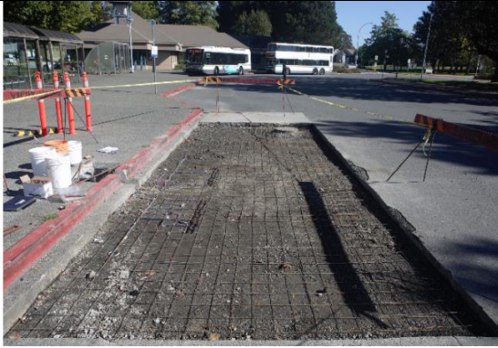
a) Excavated Site laid with wire mesh
