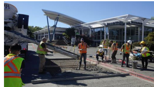
f) Concrete pour from truck directly mixed with fibers
