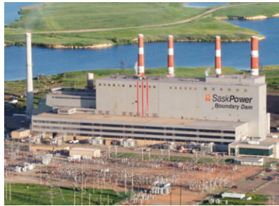
Boundary Dam Power Station
