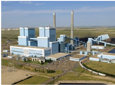
Antelope Valley Station
