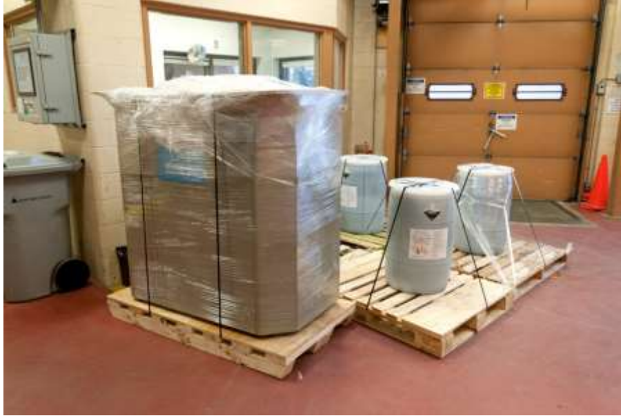
Figure 1 - VRB arrival in December 2017 at Shell Technology Centre Calgary
