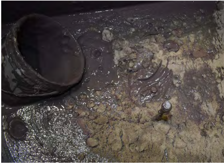
Figure 23 VW-6 Excavation during Decommissioning
