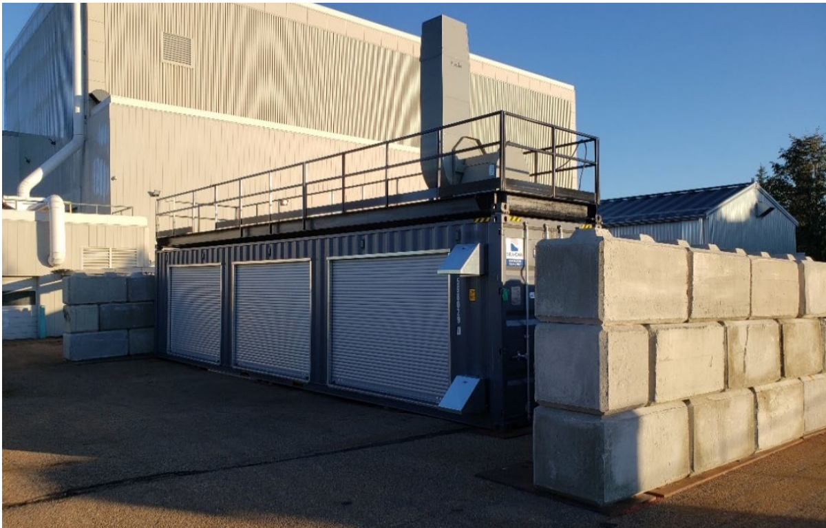
Figure 3.2 ICD Solvent Testing Facility
