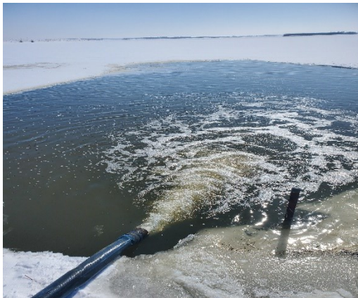
Figure 3: Demonstration of concentrate from SLU adding aeration to lagoon
