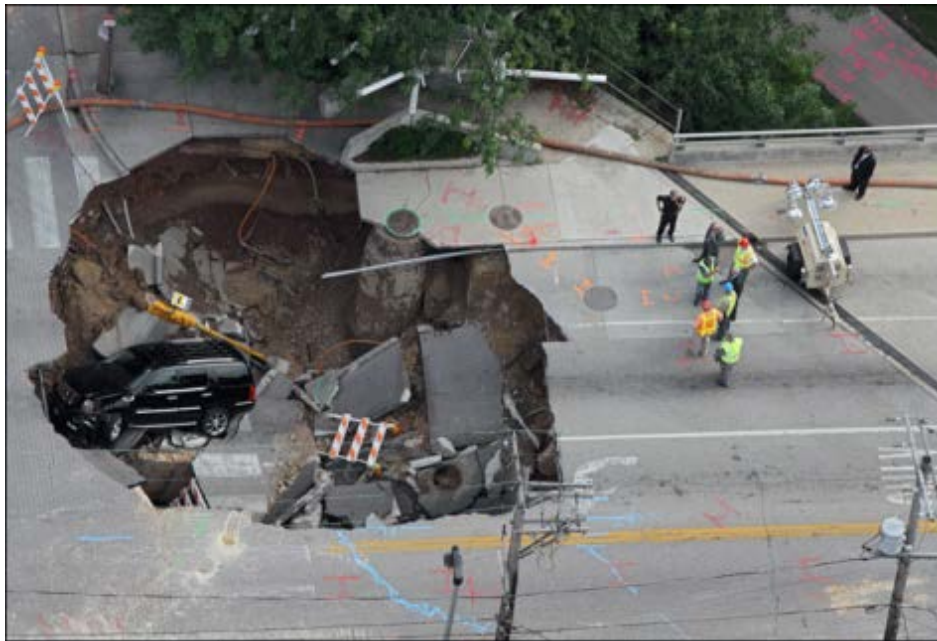
Consequences of catastrophic pipe failure. A common occurrence due to the aging water and sewer infrastructure.
