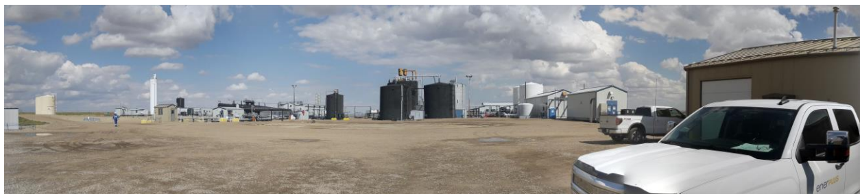
Figure 10: Pilot Plant Site
