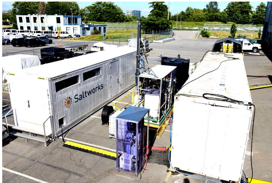
Figure 3. Pilot plant exterior
