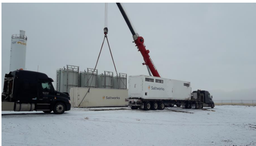
Figure 8: Pilot Plant Unloading at Site
