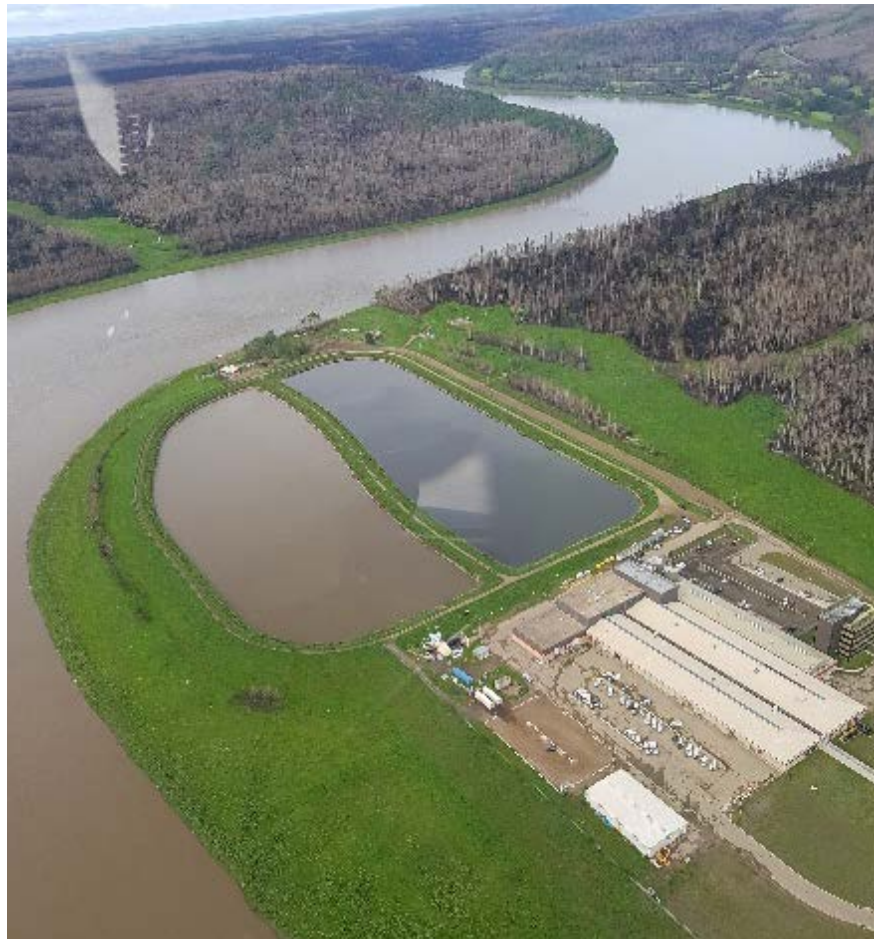
Figure 13. Aerial view of dual-stage, in-line reservoir at the RMWB's Fort McMurray WTP indicating reduction of suspended solids within the reservoir. Higher levels of suspended solids are seen in the east basin (left) closer to the river and substantial settling of suspended sediment is evident in the west basin (right).
