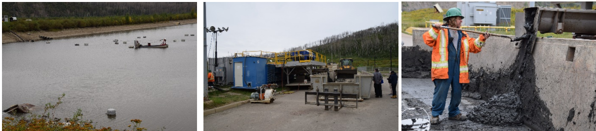
Figure 30. Dredging of the RMWB's raw water storage reservoir (west cell) at the Fort McMurray WTP in August 2018 (left). Water extraction by centrifugation to reduce sediment mass by approximately 40% (center). Collection of dewatered bottom sediment for landfill disposal (right). The process of reservoir dredging continued for approximately four months.
