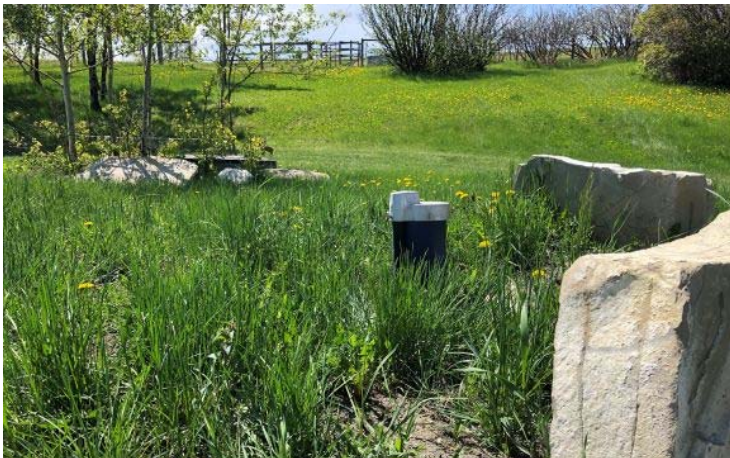
Well head on rural property. Photo S. Checkley
